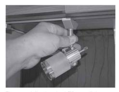
Fig. 183: Adjusting the LED spot light
