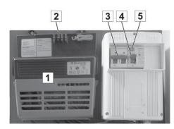
Fig. 61: Converter (power supply unit) (1) and cut-outs
