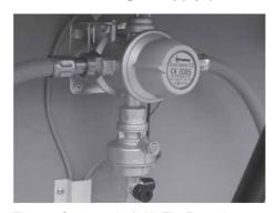
Fig. 76: Gas supply (with Eis-Ex and remote control)
