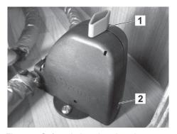
Fig. 108: Safety drain valve closed
