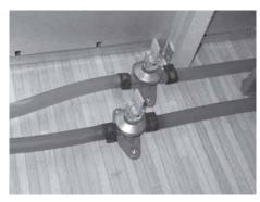
Fig. 100: Drain valves opened
