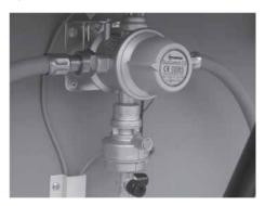
Fig. 114: DuoControl CS gas supply
