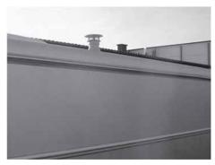
Fig. 82: Exhaust gas stack of the gas heater
