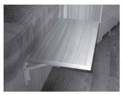
Fig. 181: Folding console as bed extension
