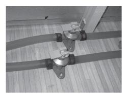
Fig. 176: Closed drain valves
