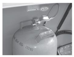
Fig. 112: Gas bottle with pressure reducing valve
