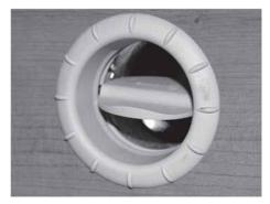
Fig. 133: Hot-air nozzle, open
