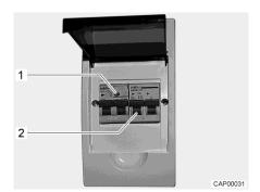
Fig. 47 230 V fuse box with safety cut-out and FI-switch
