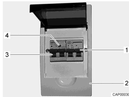
Fig. 42 Safety cut-out and FI-switch (230 V fuse box)
