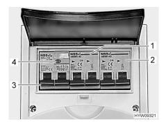
Fig. 115 Safety cut-out and FI-switch (230 V fuse box)
