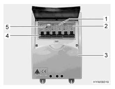
Fig. 110 Safety cut-out and FI-switch (230 V fuse box)
