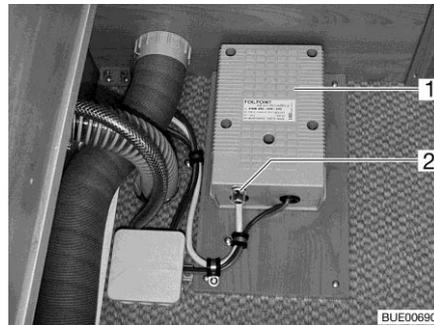
Fig. 120 Transformer for electrical floor warming unit
