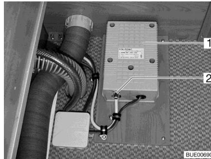
Fig. 244 Transformer for electrical floor warming unit
