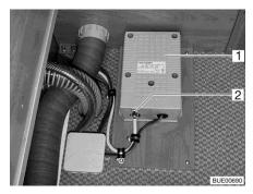
Fig. 120 Transformer for electrical floor warming unit
