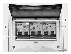
Fig. 107 Safety cutout and FI-switch (230 V fuse box)
