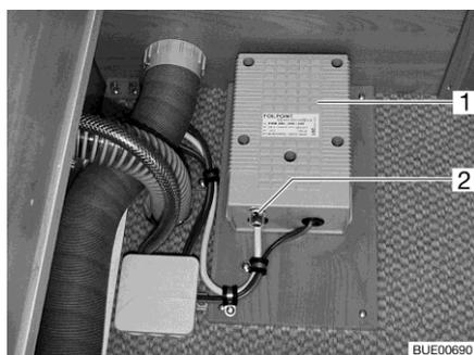
Fig. 226 Transformer for electrical floor warming unit
