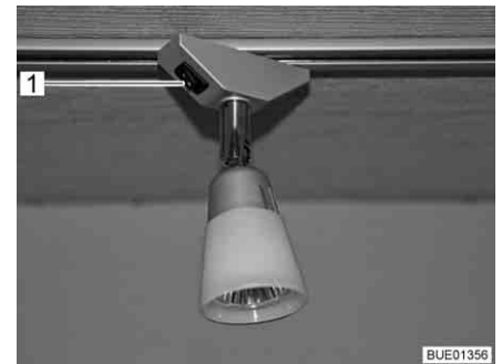
Fig. 62 Halogen spotlight, light switch directly on the lamp
