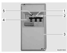
Fig. 143 230 V fuse box with safety cutout and FI-switch
