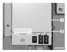
Fig. 150 Heater regulation for waste water pipes
