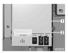
Fig. 167 Heater regulation for waste water pipes
