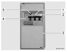
Fig. 168 230 V fuse box with safety cutout and FI-switch
