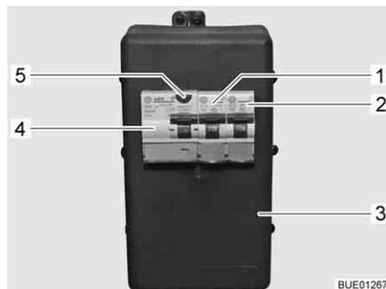
Fig. 142 230 V fuse box with safety cut-out and FI-switch
