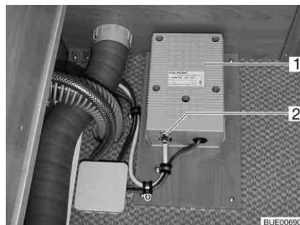
Fig. 211 Transformer for electrical floor warming unit
