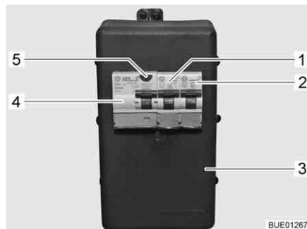
Fig. 189 230 V fuse box with safety cut-out and FI-switch
