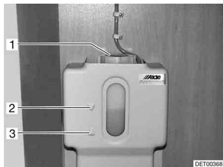
Fig. 289 Compensator reservoir hot-water heater
