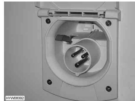
Fig. 124 230 V connection on vehicle
