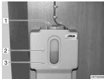
Fig. 219 Compensator reservoir hot-water heater
