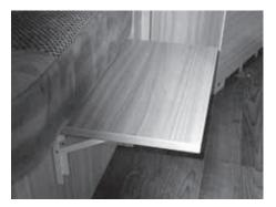
Fig. 129: Folding console as bed extension
