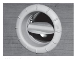
Fig. 77: Hot-air nozzle, open
