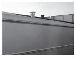
Fig. 78: Exhaust gas stack of the gas heater
