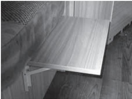
*Fig. 129: Folding console as bed extension*
