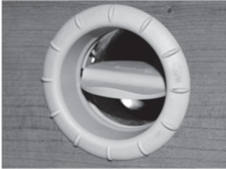
Fig. 118: Hot-air nozzle, open
