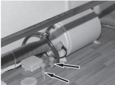
Fig. 121: Drain valves
