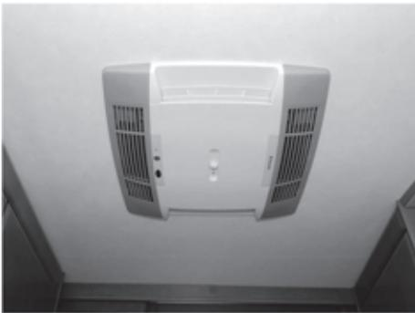
Fig. 27: Air conditioning system (optional)
