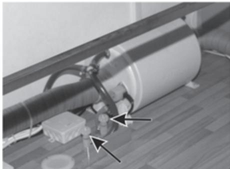
Fig. 86: TRUMA water heating and water drain valves
