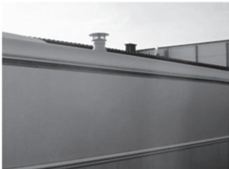
Fig. 78: Exhaust gas stack of the gas heater
