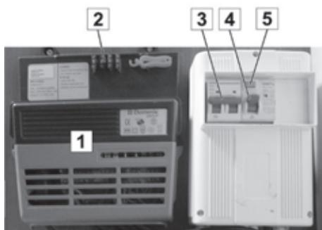
Fig. 58: Converter (power supply unit) (1) and cut-outs
