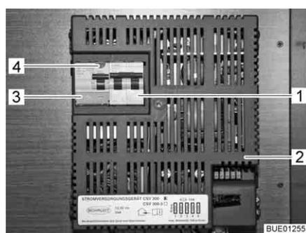
Fig. 124 230 V fuse box with safety cut-out and FI-switch
