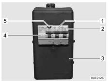
Fig. 99 230 V fuse box with safety cutout and FI-switch
