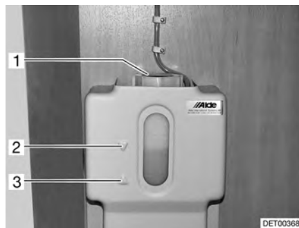
Fig. 199 Compensator reservoir hot-water heater
