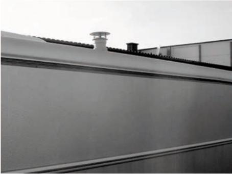
Fig. 85: Exhaust gas stack of the gas heater
