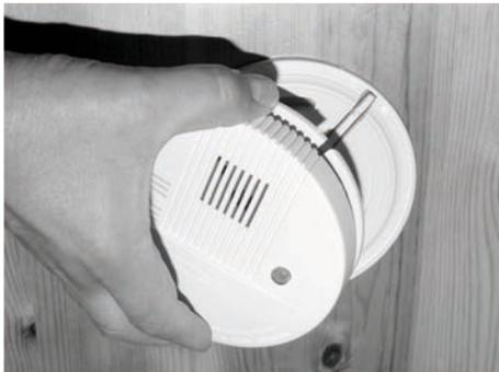
Fig. 110: Removing the housing
