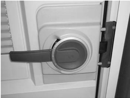
Fig. 20: Closed but unsecured door lock
