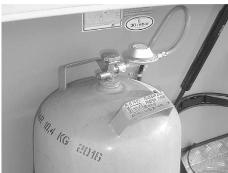
Fig. 103: Gas bottle with pressure reducing valve
