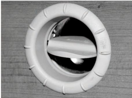
Fig. 128: Hot-air nozzle, open
