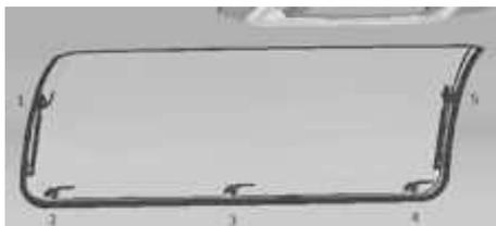
Fig. 37: Inside view of the domed hinged window with five sash fasteners
