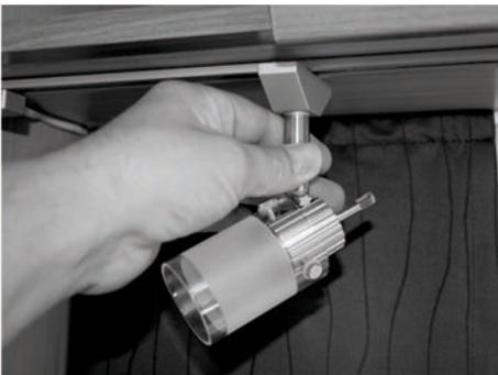
Fig. 140: Adjusting the LED spot light
