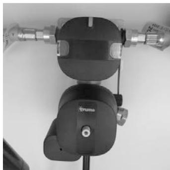
Fig. 105: DuoControl CS gas supply
