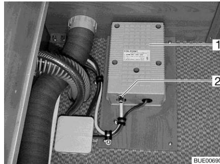
Fig. 233 Transformer for electrical floor warming unit
