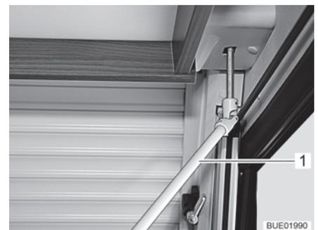
Fig. 106 Hand crank for emergency operation
