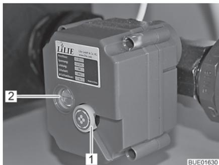
Fig. 196 Electrically operated drainage valve
