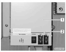
Fig. 115 Heater regulation for waste water pipes
