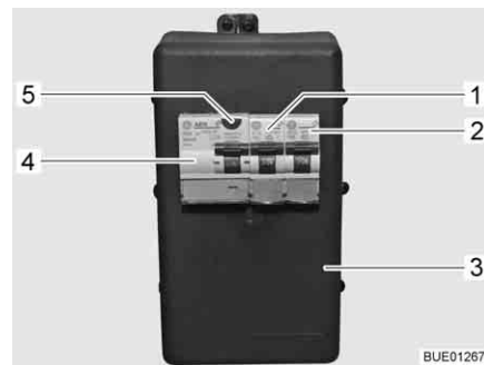
Fig. 160 230 V fuse box with safety cut-out and FI-switch
