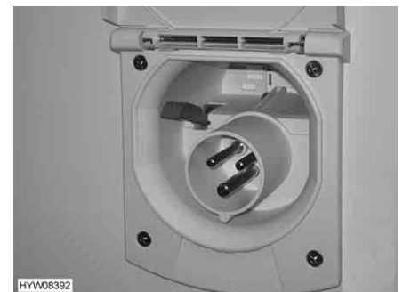
Fig. 161 230 V connection on vehicle
