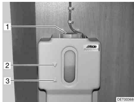
Fig. 254 Compensator reservoir with panel
