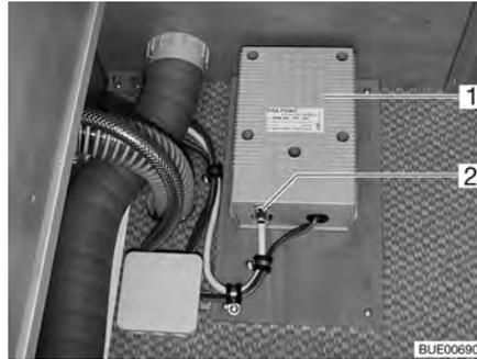
Fig. 166 Transformer for electrical floor warming unit
