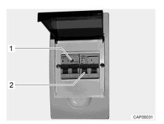
Fig. 76 230 V fuse box with safety cut-out and FI-switch
