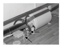
Fig. 93: TRUMA water heating and water drain valves
