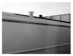
Fig. 85: Exhaust gas stack of the gas heater
