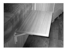
Fig. 138: Folding console as bed extension
