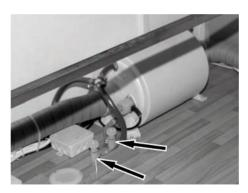
Fig. 131: Drain valves
