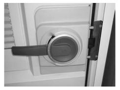
Fig. 20: Closed but unsecured door lock
