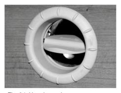
Fig. 84: Hot-air nozzle, open
