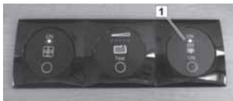
Fig. 83: On-Off switch of the floor heating system
