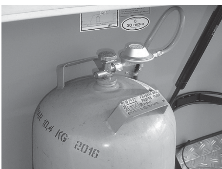
Fig. 114: Gas bottle with pressure reducing valve
