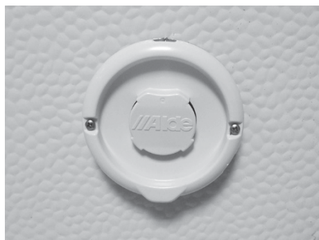
Fig. 88: Wall exhaust stack
