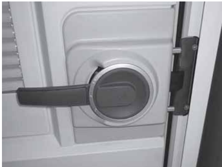
Fig. 13: Closed but unsecured door lock
