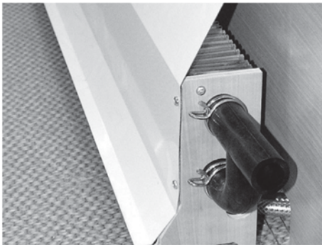
Fig. 90: Convector with thermally conductive panel
