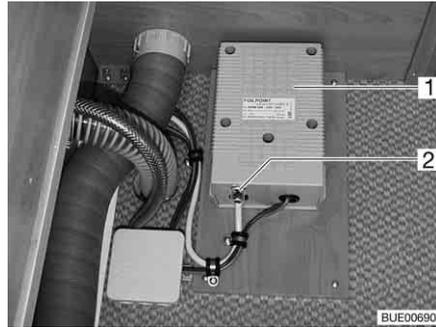
Fig. 131 Transformer for electrical floor warming unit
