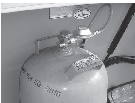
Fig. 101: Gas bottle with pressure reducing valve
