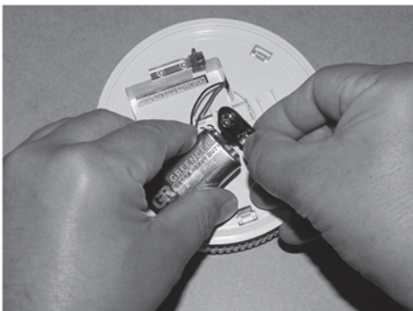
Fig. 109: Replacing the block battery
