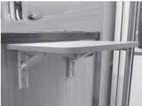
Fig. 200: Folding console to extend the kitchen counter-top
