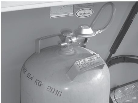
Fig. 112: Gas bottle with pressure reducing valve
