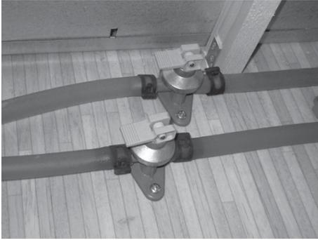
*Fig. 176: Closed drain valves*
