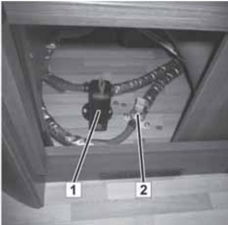
Fig. 106: TRUMA combination heater drain valves
