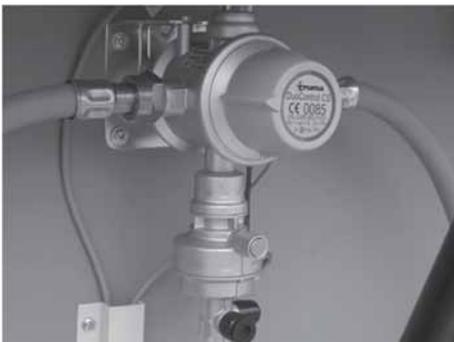
Fig. 114: DuoControl CS gas supply
