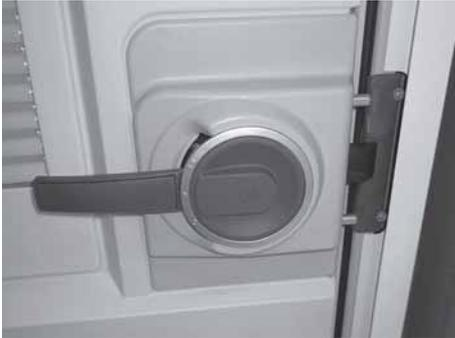
Fig. 13: Closed but unsecured door lock
