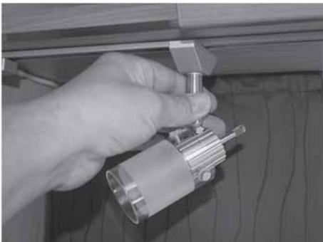
Fig. 183: Adjusting the LED spot light
