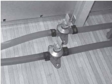
Fig. 100: Drain valves opened
