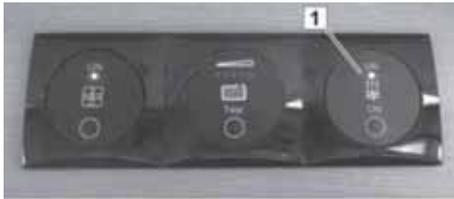
Fig. 134: On-Off switch of the floor heating system
