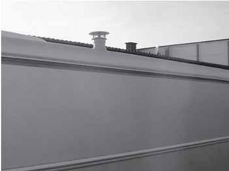
Fig. 82: Exhaust gas stack of the gas heater
