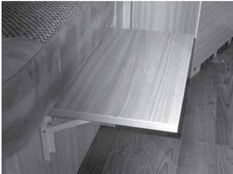
Fig. 181: Folding console as bed extension
