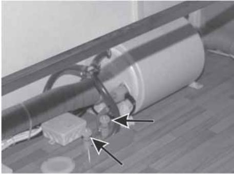
Fig. 97: TRUMA water heating and water drain valves
