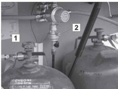
Fig. 116: Gasstrykkregulator
