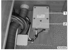
Fig. 211 Transformer for electrical floor warming unit
