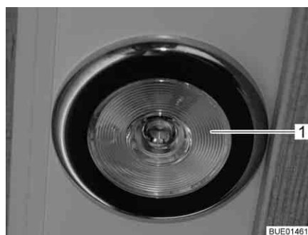
Fig. 69 Recessed light, light switch in the lamp
