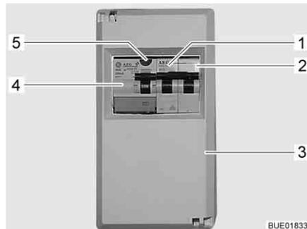
Fig. 161 230 V fuse box with safety cut-out and FI-switch
