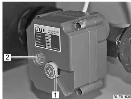
Fig. 230 Electrically operated drainage valve
