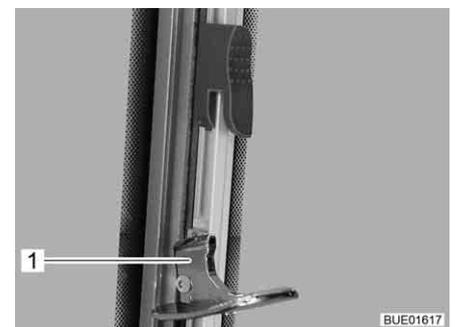
Fig. 109 Sliding window with swivel lock (unlocked)
