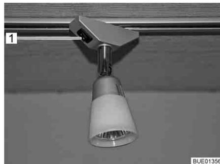
Fig. 45 Spotlight, switch mounted directly on the lamp
