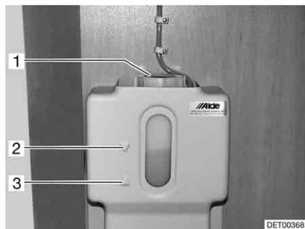
Fig. 196 Compensator reservoir hot-water heater
