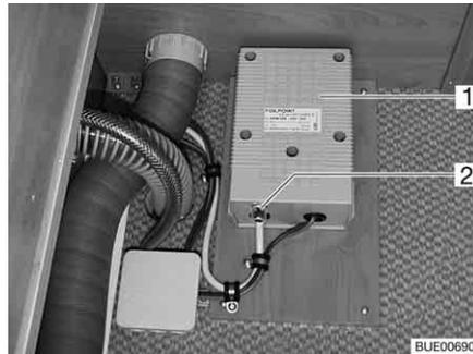
Fig. 186 Transformer for electrical floor warming unit
