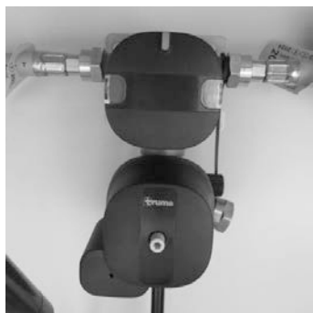
Fig. 105: Suministro de gas DuoControl CS
