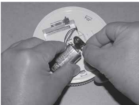
Fig. 94: Replacing the block battery
