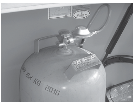
Fig. 92: Gas bottle with pressure reducing valve
