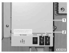
Fig. 129 Heater regulation for waste water pipes
