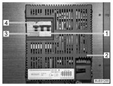
Fig. 130 230 V automatic circuit breaker and FI-switch (CSV 300)
