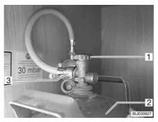
Fig. 116 Gas bottle compartment
