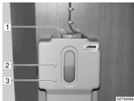
Fig. 212 Compensator reservoir with panel
