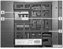
Fig. 121 230 V fuse box with safety cutout and FI-switch
