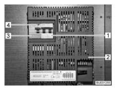
Fig. 126 230 V automatic circuit breaker and FI-switch (CSV 300)
