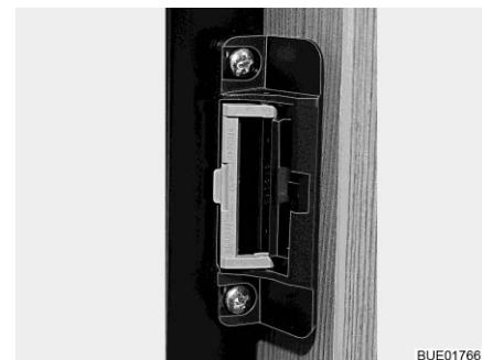
Fig. 246 Locking device in ventilation position
