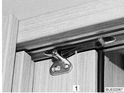
Fig. 17 Catch with spring
