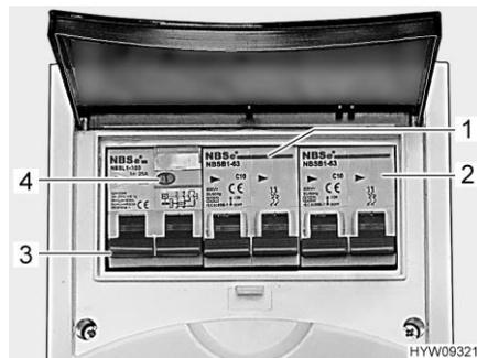
Fig. 121 Safety cut-out and FI-switch (230 V fuse box)
